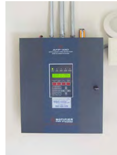
Typical building-based fire alarm control panel – Management reports widespread operational issues
