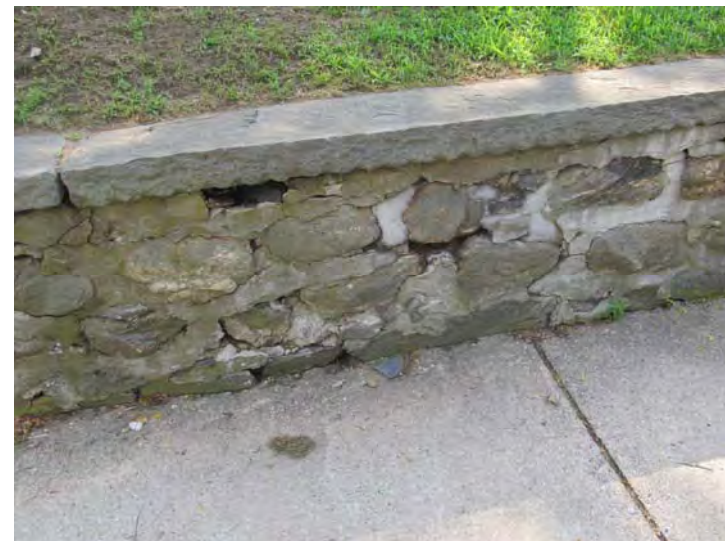
Stone retaining wall located at street, along front of site, is in need of selective repairs
