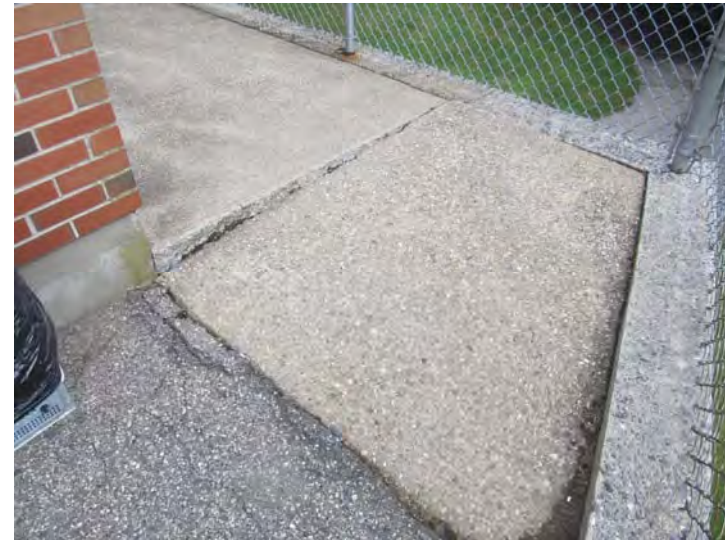
Cracks and displacement at pedestrian walkways present potential trip hazards
