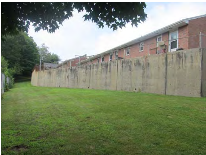
Large poured concrete retaining wall located behind Buildings A and B is in generally good condition
