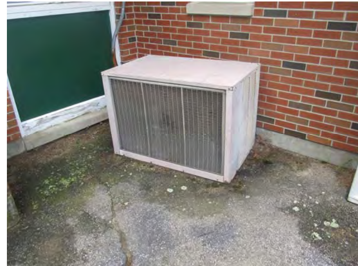
Exterior, air-cooled, condenser unit for cooling at community room is surpassed its expected useful service life
