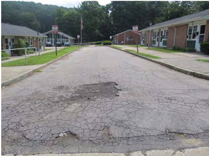
Asphalt-paved access and parking area surfaces exhibit wear and damage
