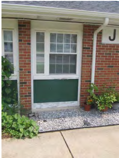
Infill panels under windows exhibits wear
