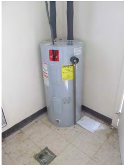
Electric-type domestic hot water tank serving the community building
