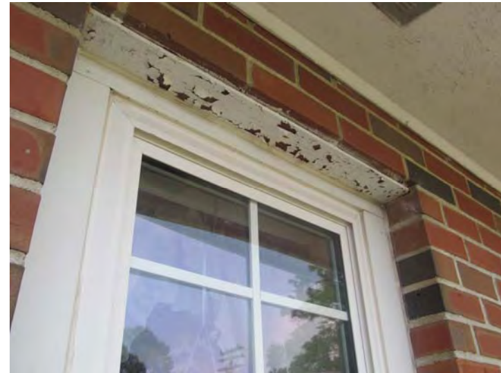
Steel lintels over windows set in masonry openings are in need of surface preparation and painting
