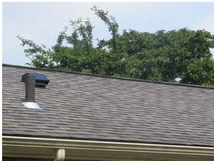
Architectural shingles were installed on all roof surfaces at the development in recent years
