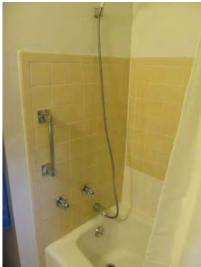
Original, multi-stem, mixing valve assemblies are typical at unit bathtubs
